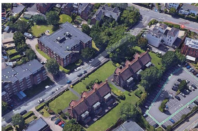
Grendon Road Almshouses, 4th Remodelling Project to be undertaken by Exeter Homes Trust
